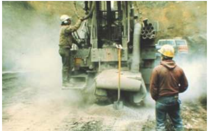
Dry Drilling in Sandstone
