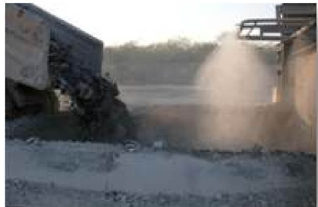
Water spraying on crusher dump hopper
