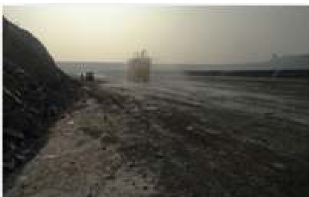
Dust suppression on Haul Road
